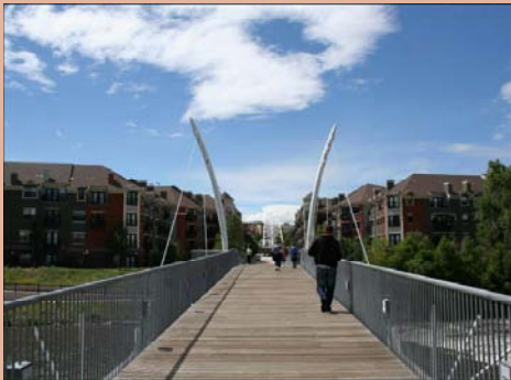
multi-use path bridges across freeways and creeks
