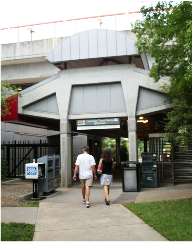
Riders entering the Dunwoody MARTA station. Photo credit: Lose & Associates, Inc.
